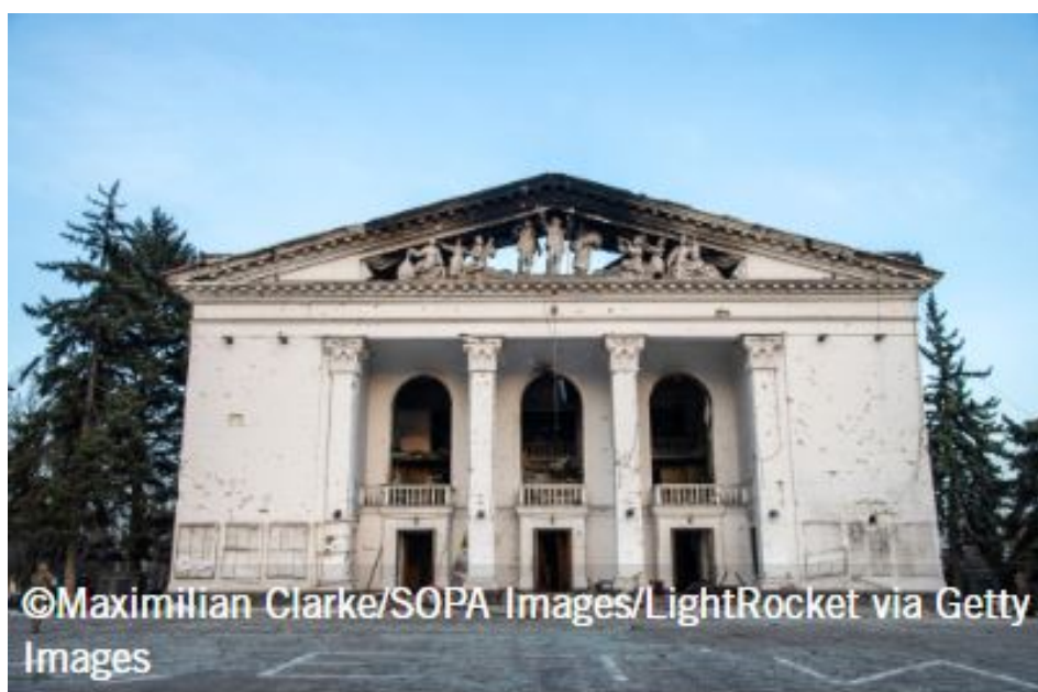
The damaged Drama Theatre in Mariupol, with the word 'children' clearly written in the foreground.
